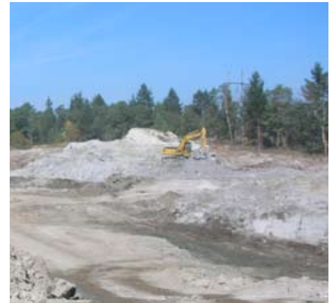
The central landfill as it approached completion of remediation in September
