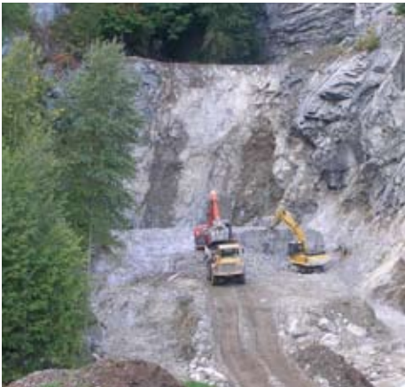
Crews finalize clean up of Bamberton's landfills early this Fall
